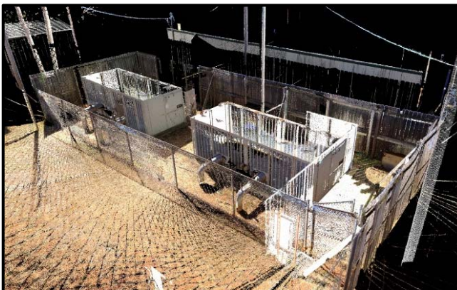
A Faro scan of the as-built conditions of two air-cooled chillers (right), and the 3D model (left).
