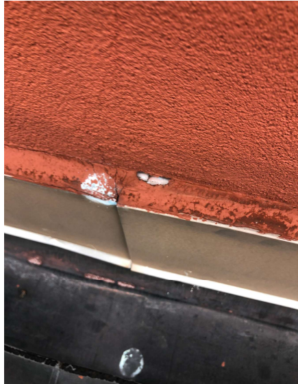
• Opening in sealants
