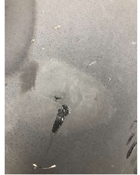
• Holes in field of roof
