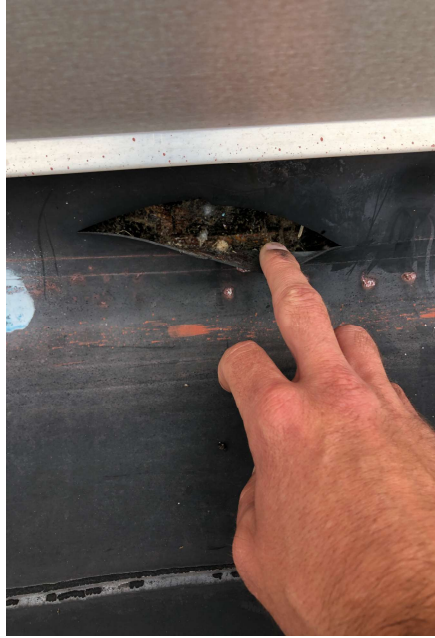
• Opening in flashings
